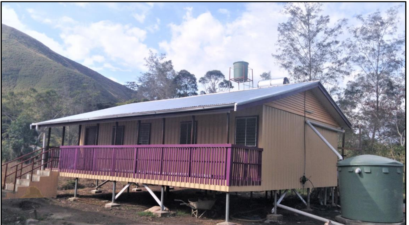
Umi Community Health Building, Dei District, Papua New Guinea Highlands, constructed during 2020 for Western Highlands Health Services Design and funding by Partner Housing (with generous individual donations), Construction by Vision for Homes (PNG)
